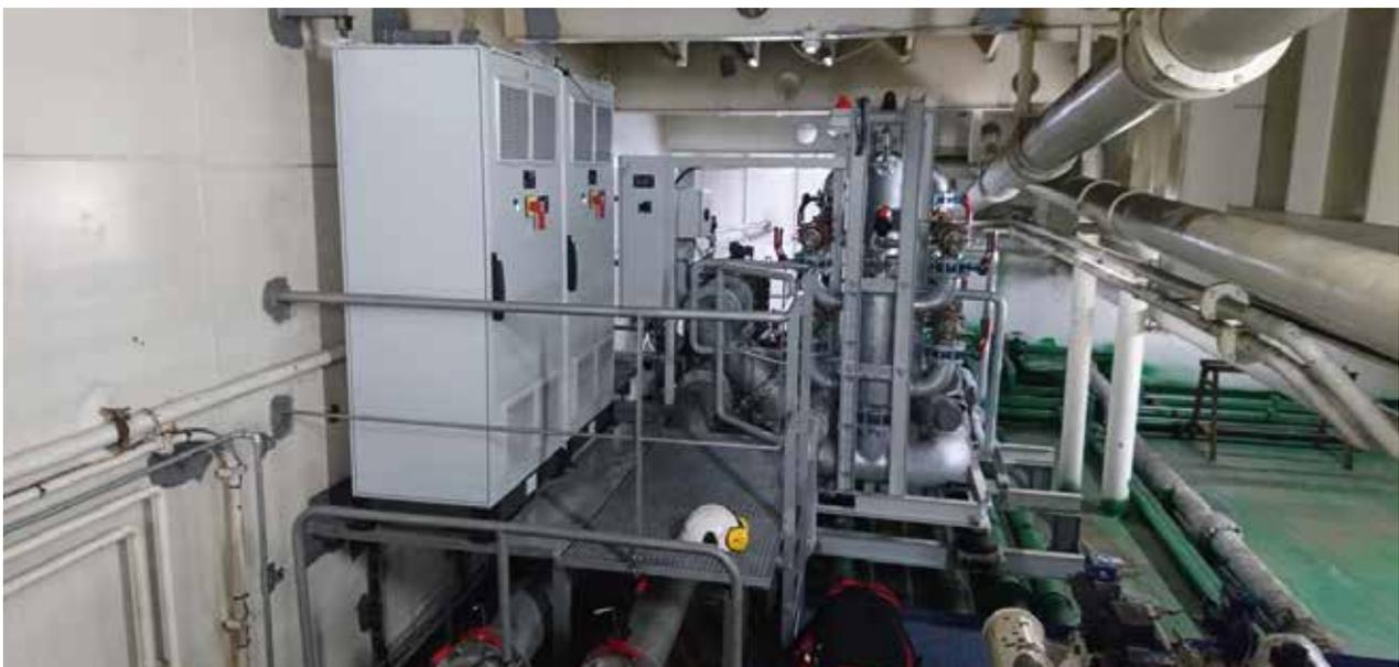
*A Bio-Sea BWTS seen installed on board ship*
